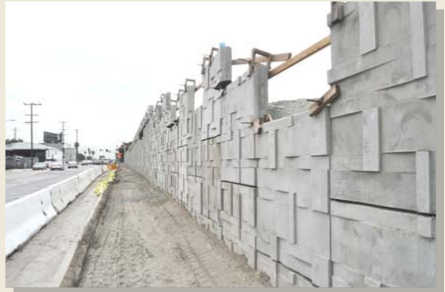
MSE wall panels west of La Cienega Boulevard
