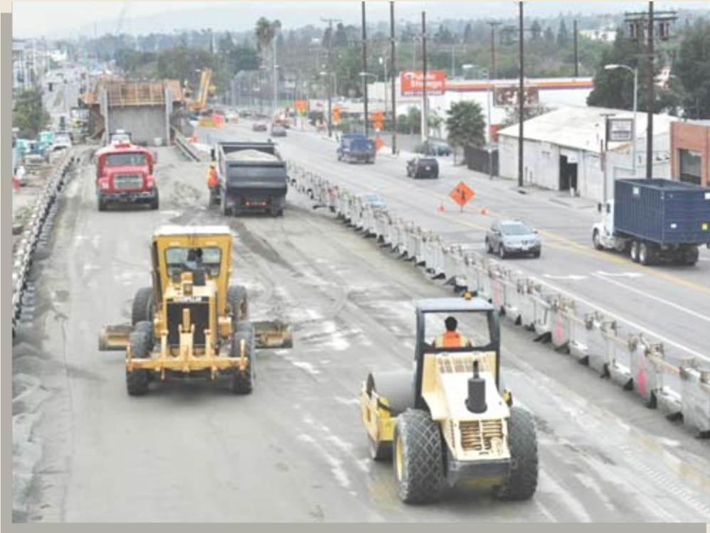
Construction of MSE walls west of La Cienega Blvd.
