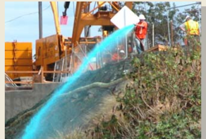
Spraying of soil binder at Jefferson Blvd
