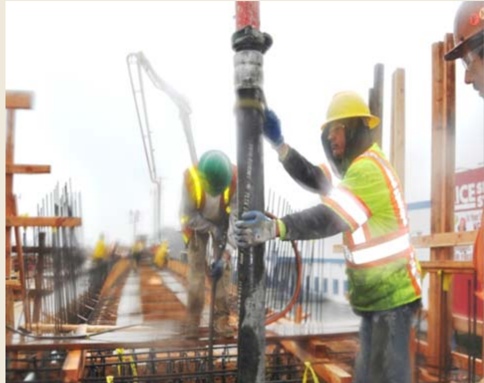
Placing of concrete at the La Brea aerial structure.
